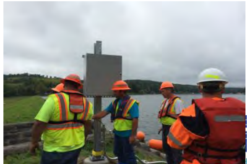
Bubbler Compressor and DCP
