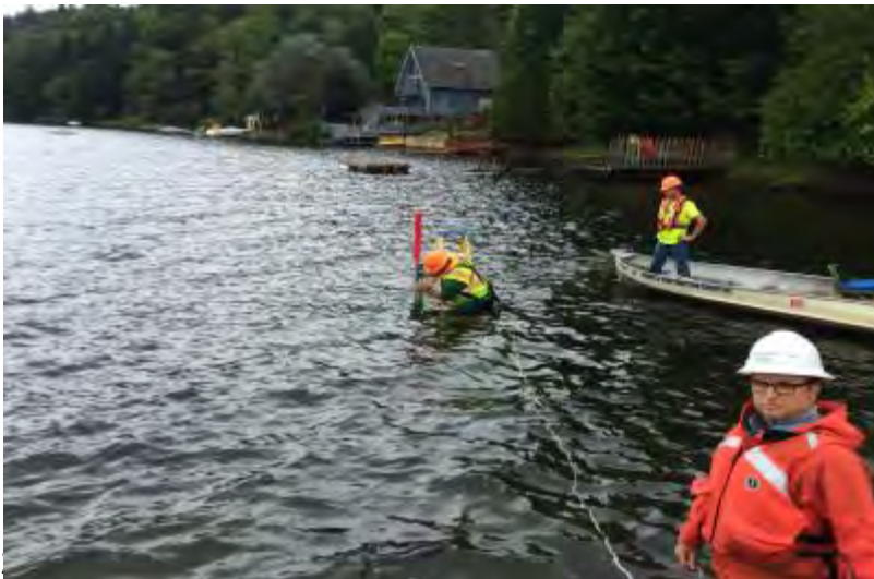
Bubbler Orifice Line Installation
