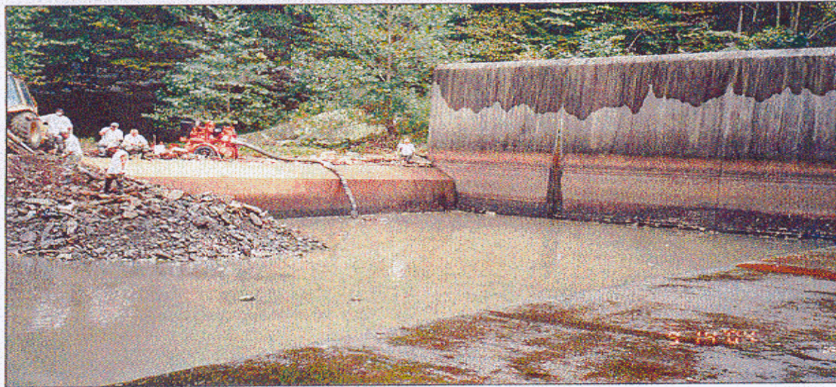
Photo 6. Stilling Basin Endsill
