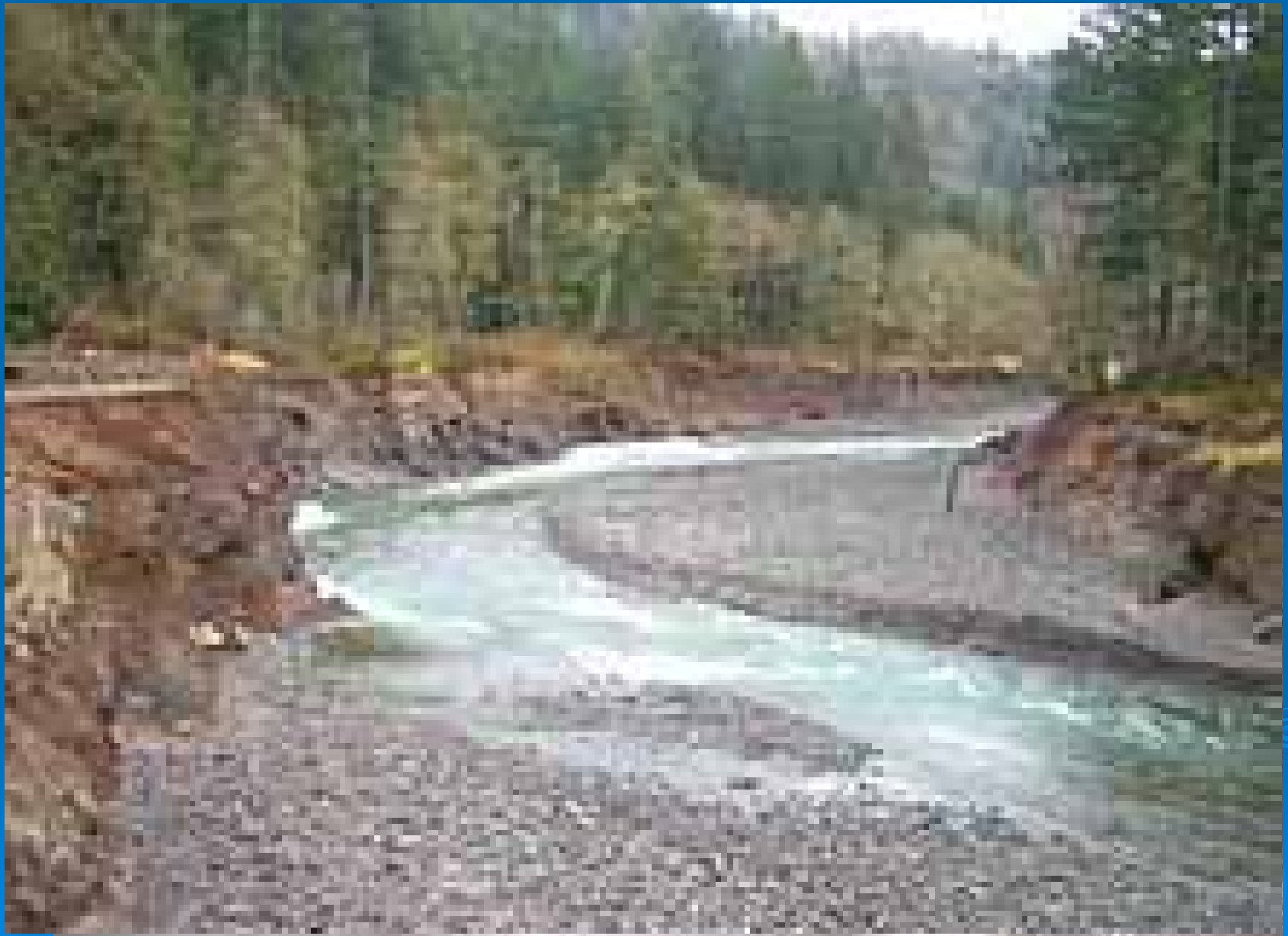
Marmot Dam Removal, Sandy River, Oregon
