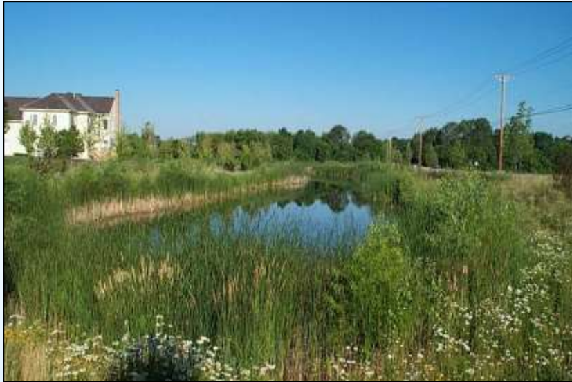
Wet Detention Basins
