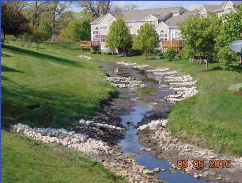
Stream Meander & Shore Stabilization
