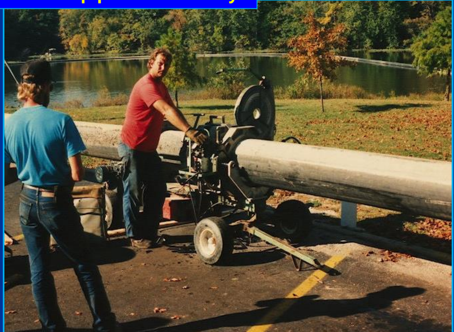
Hydraulic dredge mobilization and pipeline assembly.
