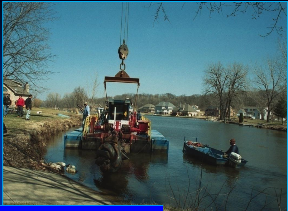
Hydraulic dredge mobilization and pipeline assembly.
