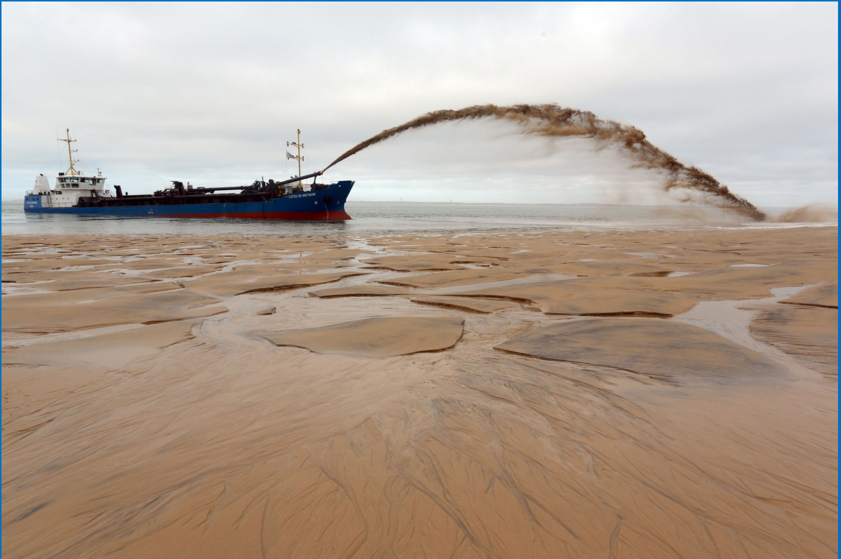
Rainbowing Dredged Sand
