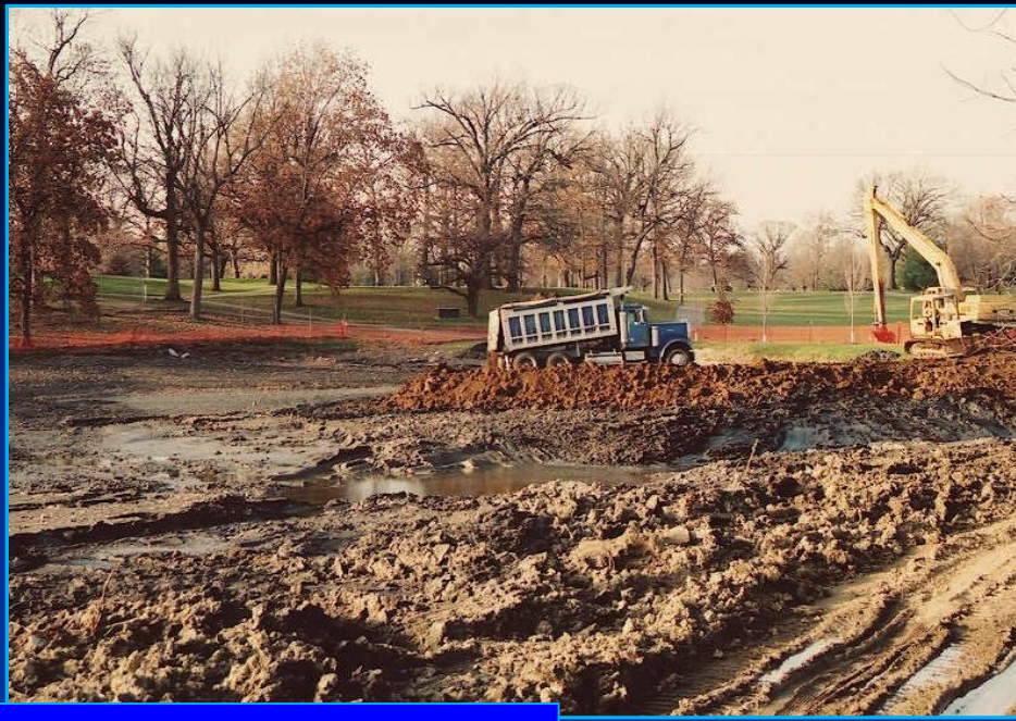
Dry Mechanical Dredging with Long Reach Excavators
