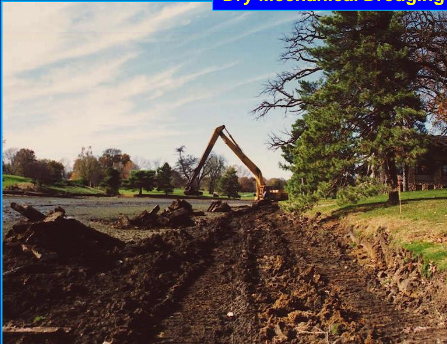
Dry Mechanical Dredging with Long Reach Excavators
