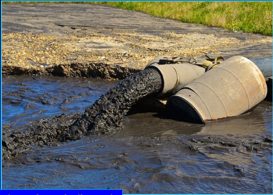
Hydraulic dredge slurry discharge from pipeline and water control structures at dewatering facilities.
