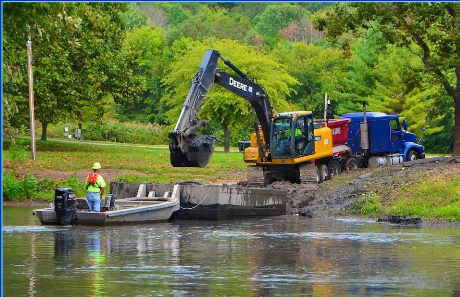
Wet Mechanical Dredging with Barge Mounted Excavators
