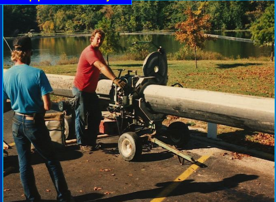
Hydraulic dredge mobilization and pipeline assembly.
