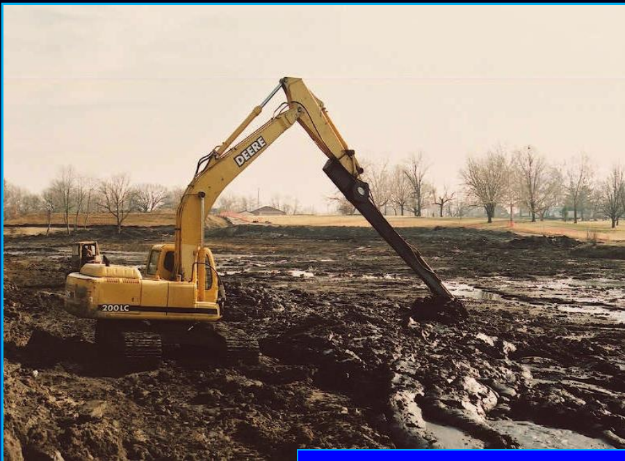
Dry Mechanical Dredging with Long Reach Excavators
