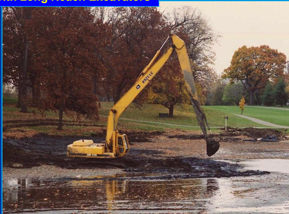
Dry Mechanical Dredging with Long Reach Excavators
