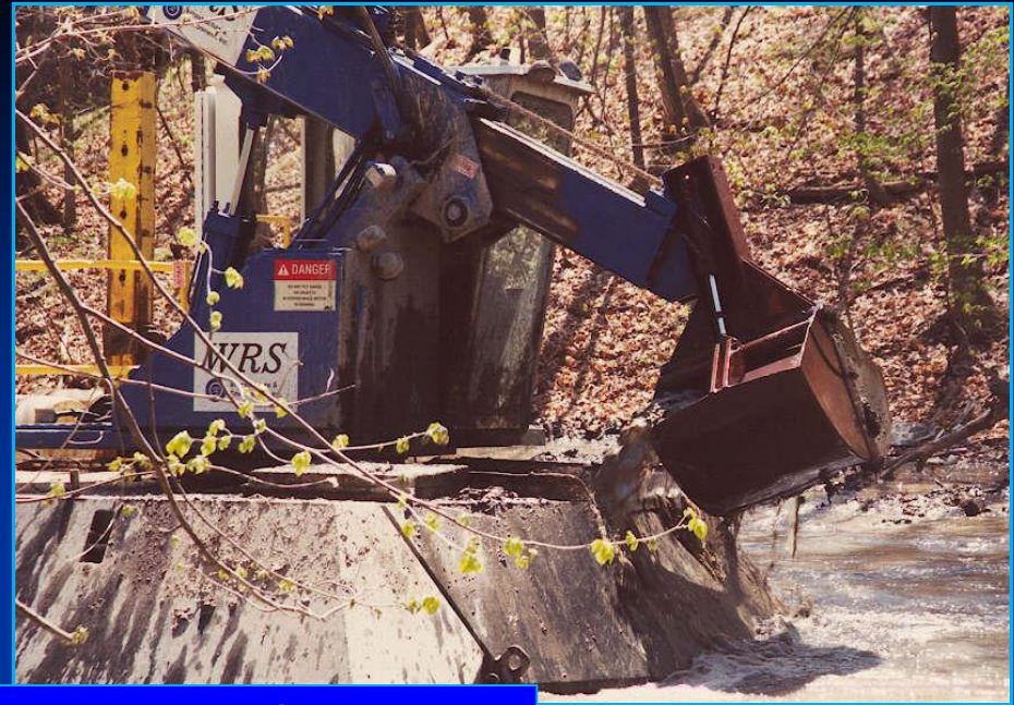
A high solids "Dry Dredge" can excavate material and pump a thickened slurry of "lava" consistency, which reduces dewatering and is efficient at filling geotextile tubes
