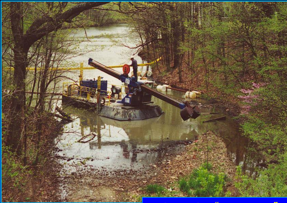
A high solids "Dry Dredge" can excavate material and pump a thickened slurry of "lava" consistency, which reduces dewatering and is efficient at filling geotextile tubes
