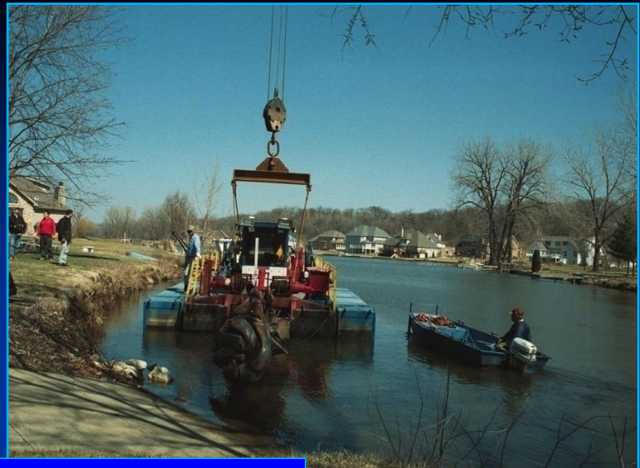
Hydraulic dredge mobilization and pipeline assembly.
