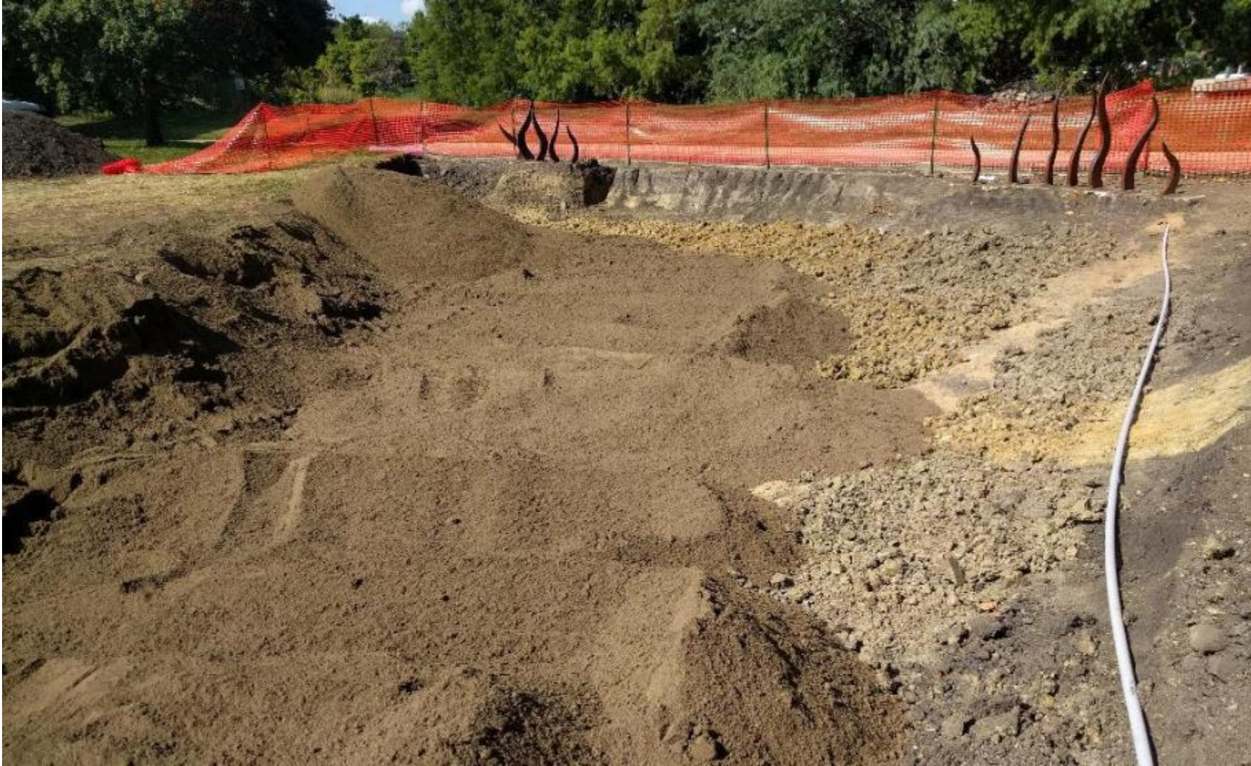
Cell 1 excavated with soil mix addition in August 2019
