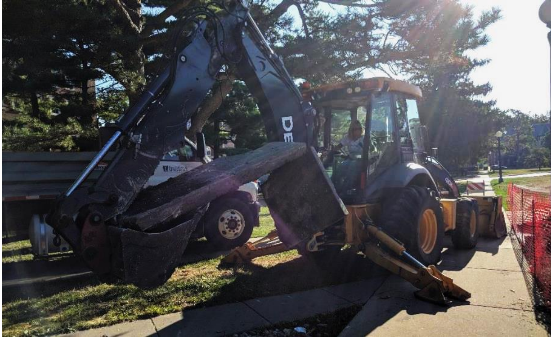
Removing the rock in August 2019
