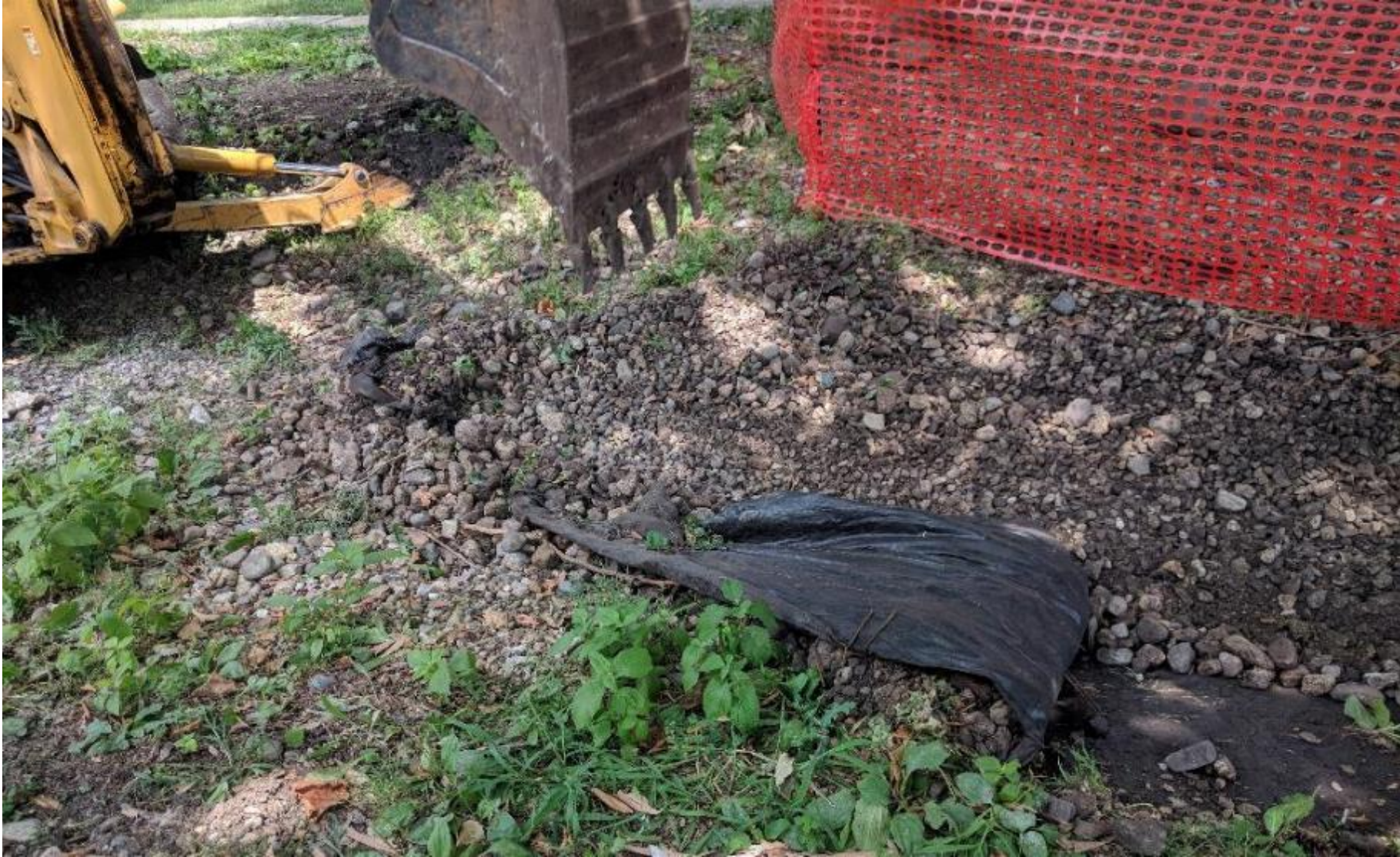
Removing the rock and landscape fabric in August 2019
