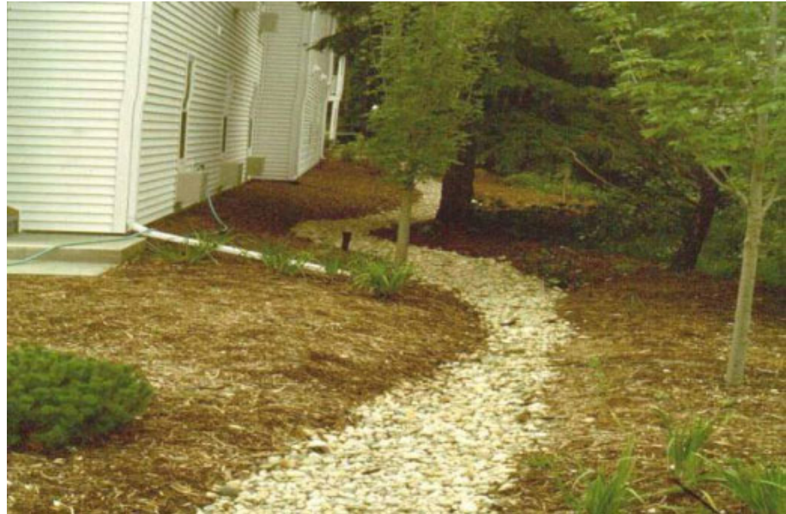
Photo provided by Chesapeake Stormwater Network
