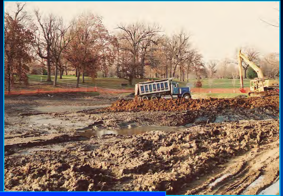
Mechanical dredging with long reach excavators at Bunn Park Lagoon
