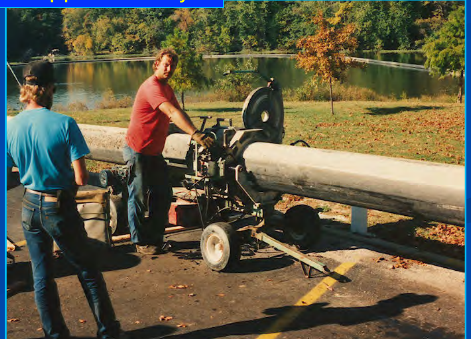
Hydraulic dredge mobilization and pipeline assembly.
