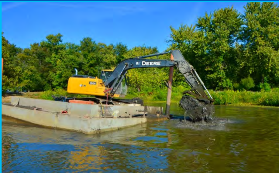
A barge mounted excavator or crane equipped with a clamshell excavating unit allows mechanical dredging in a river or waterbody without a water level drawdown.
