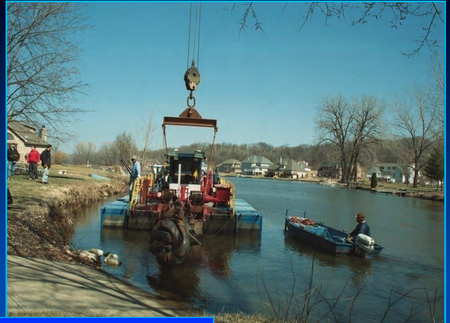
Hydraulic dredge mobilization and pipeline assembly.
