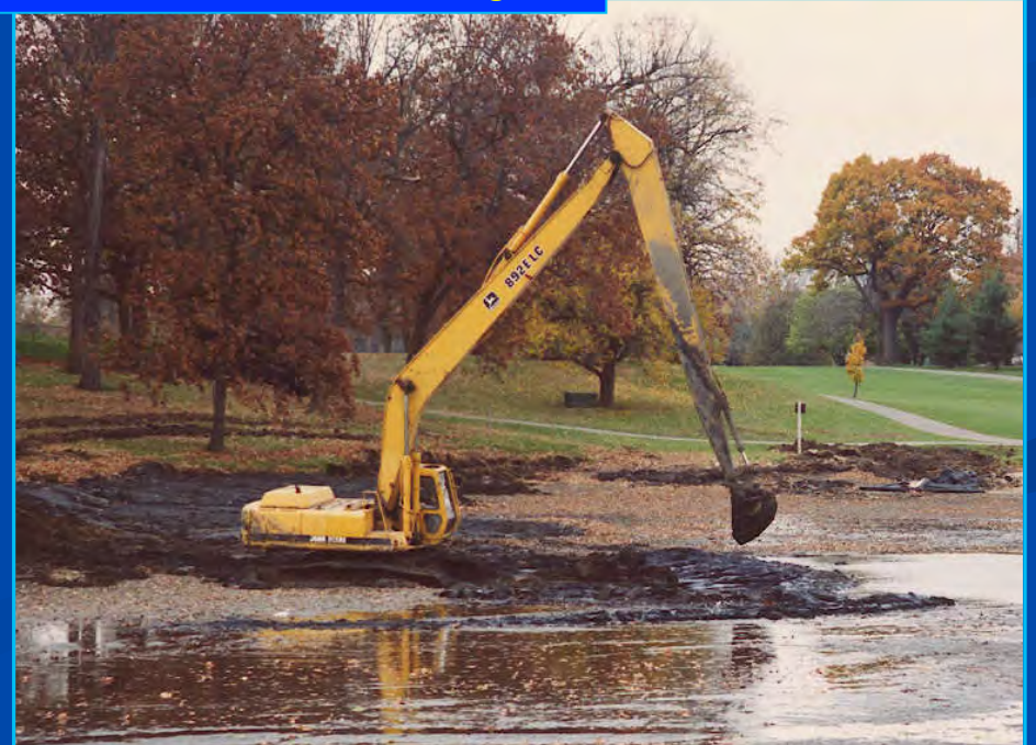
Mechanical dredging with long reach excavators at Bunn Park Lagoon
