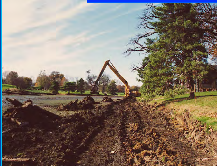
Mechanical dredging with long reach excavators at Bunn Park Lagoon
