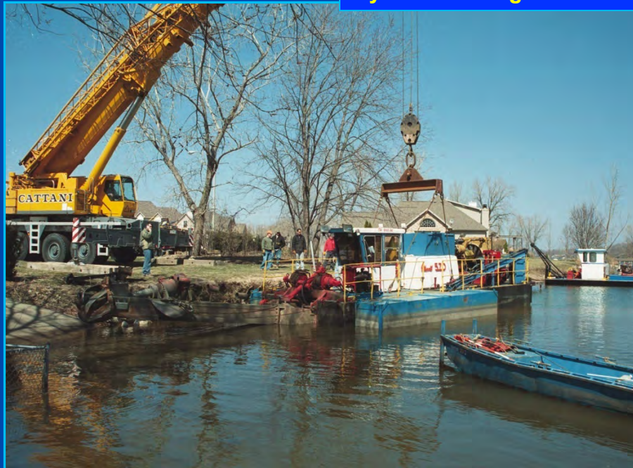
Hydraulic dredge mobilization and pipeline assembly.
