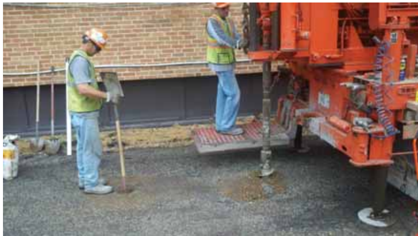
Soil boring & monitoring well installation in alley selected for permeable pavers. Measuring water level to calculate infiltration rate.
