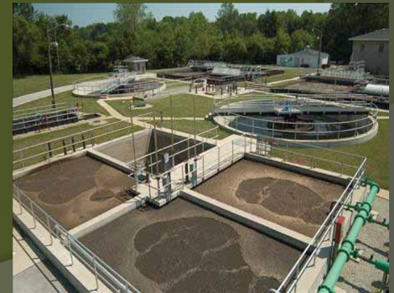
Wastewater treatment plant
