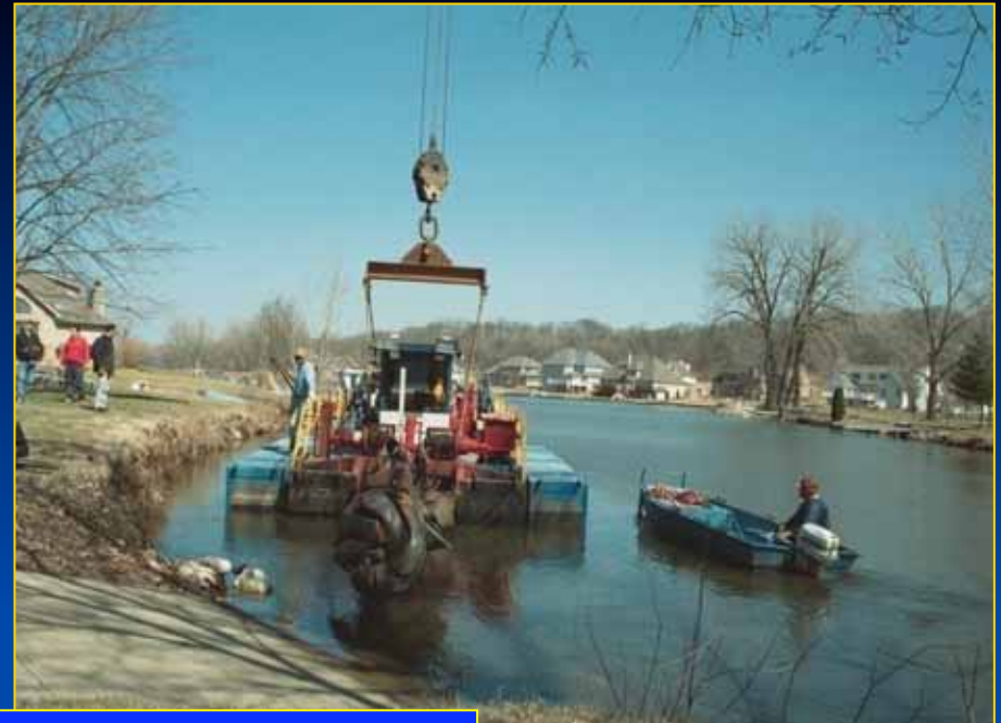
Hydraulic dredge mobilization and pipeline assembly.
