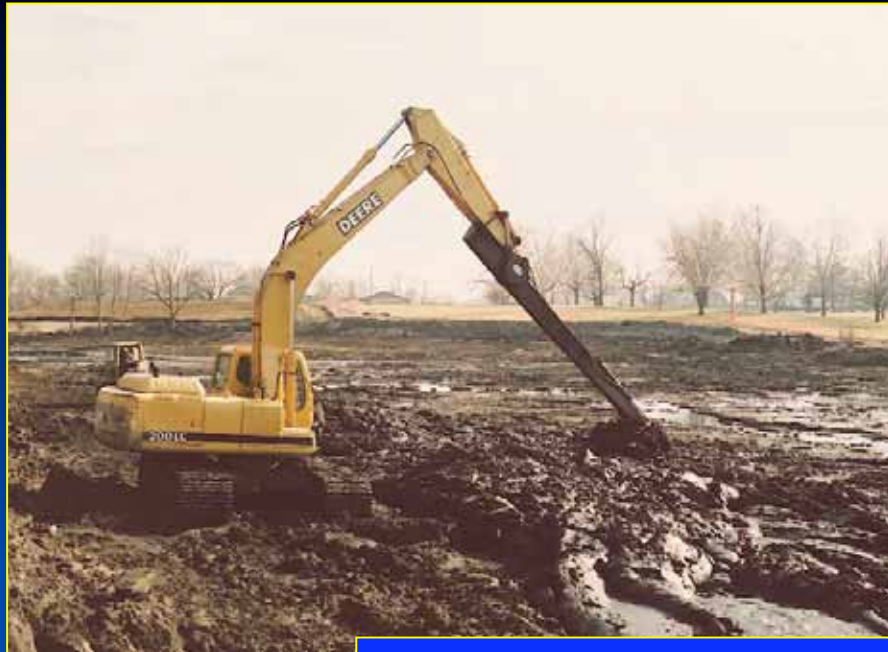
Mechanical dredging with long reach excavators at Bunn Park Lagoon
