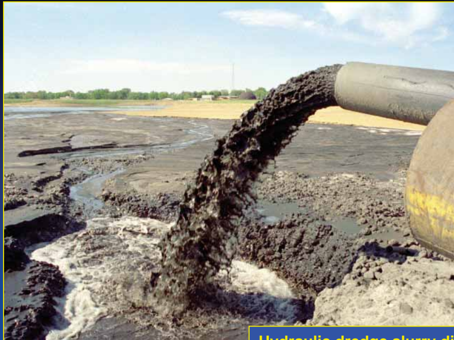
Hydraulic dredge slurry discharge from pipeline and water control structures at dewatering facilities.
