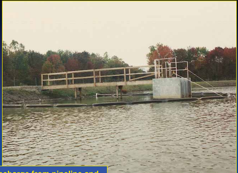
Hydraulic dredge slurry discharge from pipeline and water control structures at dewatering facilities.
