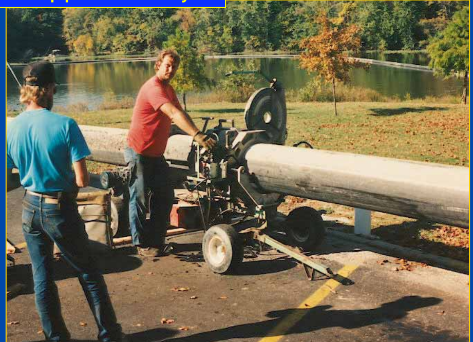
Hydraulic dredge mobilization and pipeline assembly.
