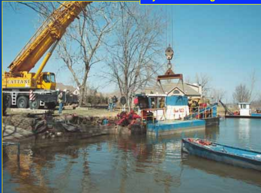
Hydraulic dredge mobilization and pipeline assembly.
