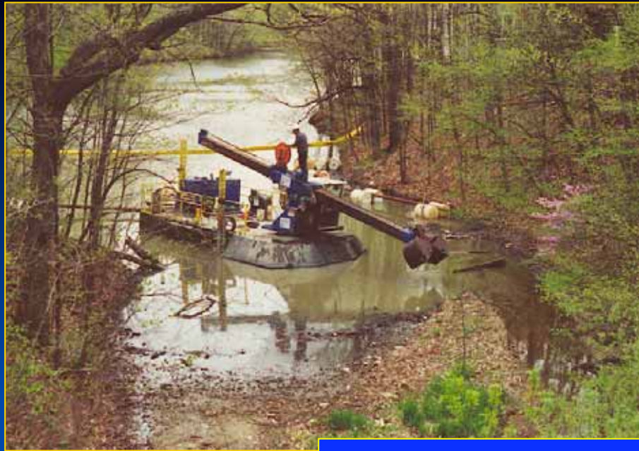
A modified high solids "Dry Dredge" can excavate material and pump a thickened slurry of "lava" consistency, which reduces dewatering and is efficient at filling geotubes.
