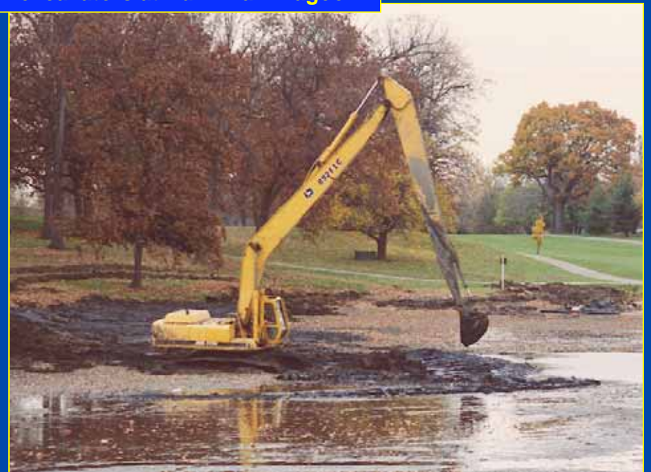
Mechanical dredging with long reach excavators at Bunn Park Lagoon
